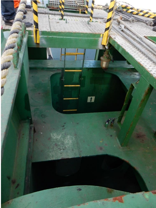
Figure 9. The cross-bay and the ladder inside of the coaming. To the right and below the ladder, i.e. on deck, the hatch to the space from where the steam is controlled. The hatch is not shown in the picture.
