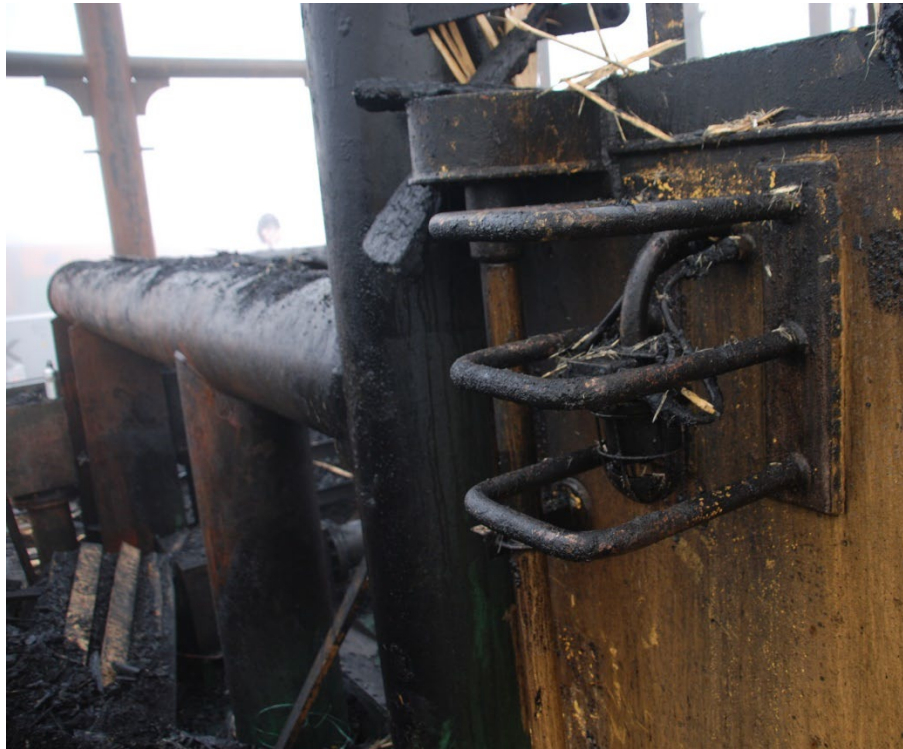
Figure 22. Fixed light fitting with protective frames on the port side deckhouse by crane 1.
