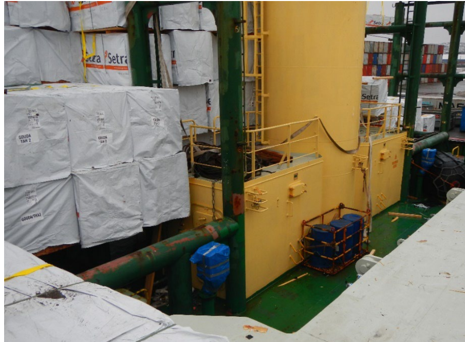
Figure 6. Lower part of crane 3 with an equivalent construction to crane 1. Deckhouses on either side of the base of the crane and the support structure with green painted pipes for the cargo to the side of the deckhouses. The accessible space under the cargo can be seen on the left of the picture.
