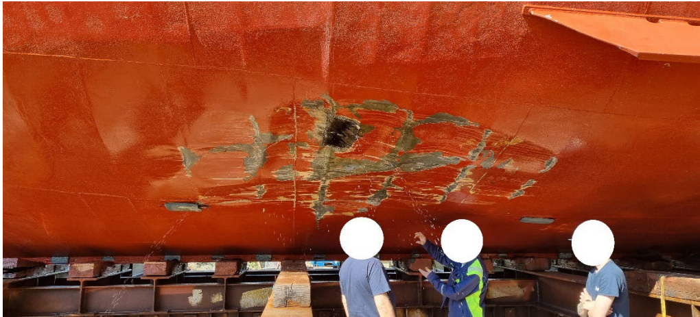
Figure 2. The picture shows the damage to the diesel tank. Photo: Rederi AB Virgo.
