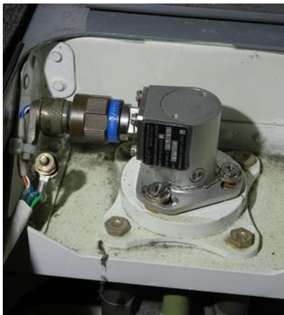
Figure 20. The sensor (RVDT) installed in the aircraft according to the installation description at the technical examination.
