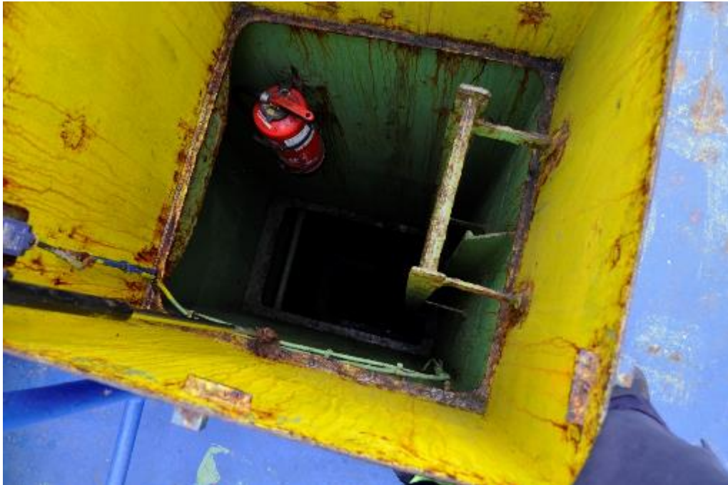
Fig. 5. The forward shaft viewed from above.
