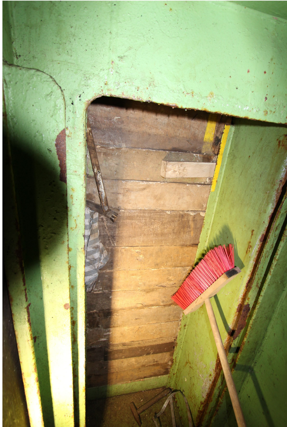
Fig. 4. The temporarily built wall in the door hole from the cargo hold shaft in to the cargo hold. The picture is taken at the bottom of the shaft and shows the inside of the door hole that is shown in Fig. 3. Image: Swedish Police Authority.
