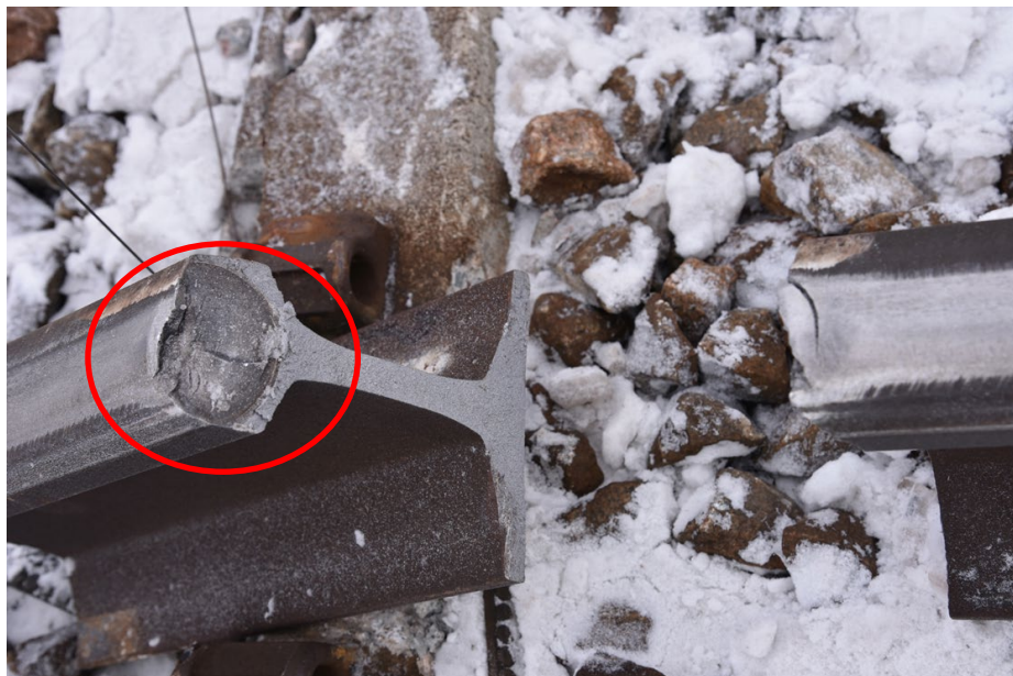
Figure 6. Signs of preceding crack formation in the rail head at the fracture surface that comes first in the direction of travel.
