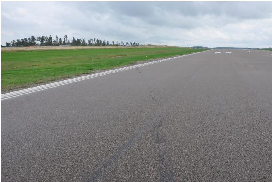
Figure 15. Clear white marks of metal and marks of rubber up to the excursion point.
