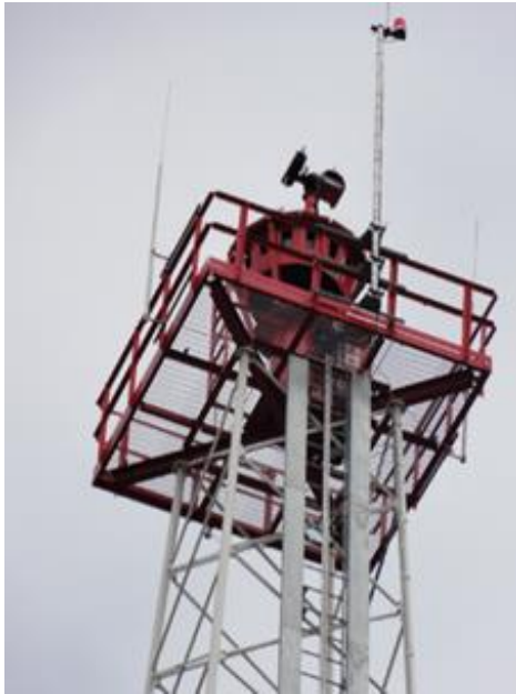
Figure 9. The camera tower at Linköping/Saab Airport.
