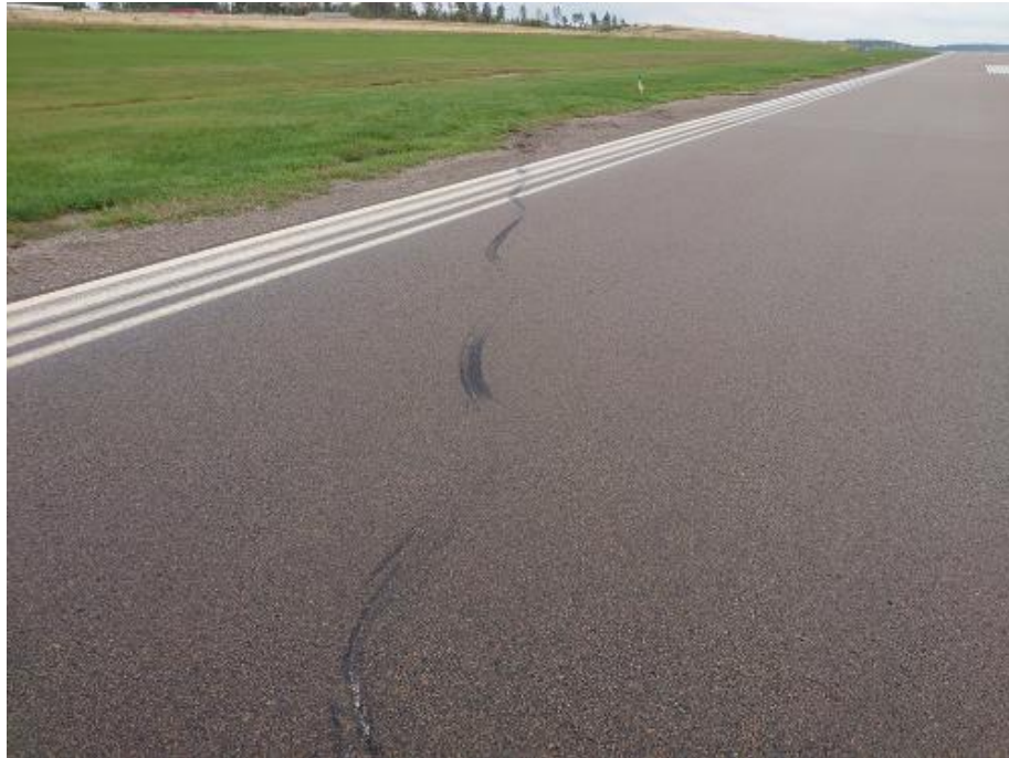
Figure 16. Marks on the runway from rubber and metal.
