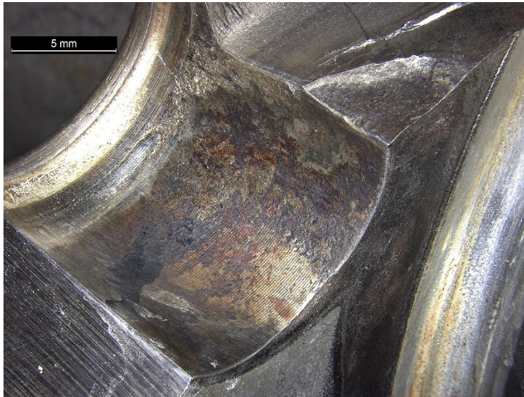
Figure 5: Corrosion observed within the bore of the dowel pin hole
