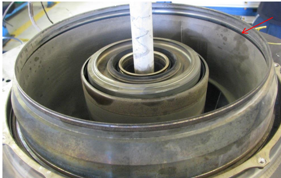
Figure 27. Rubbing damage in the turbine casing.
