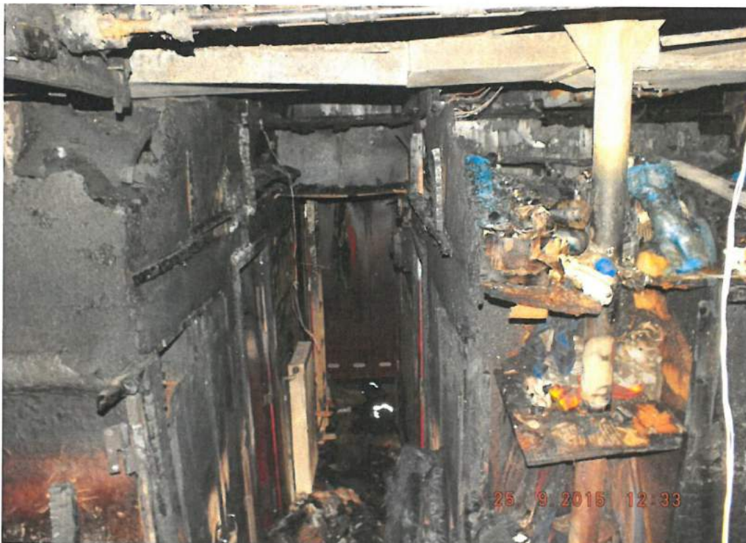
Photograph 10: The alleyway between the crew cabins
