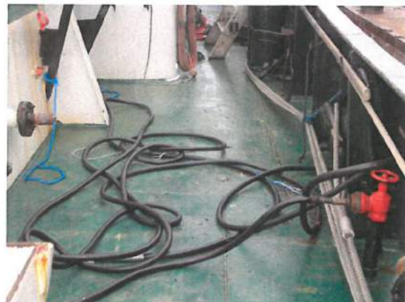
Photograph 7: A working rubber hose which was used by the crew to extinguish fire
