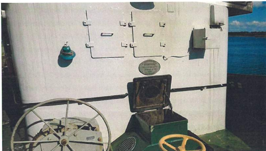
Photograph 3: The hatch in the forward deck through which the accommodation could be reached
