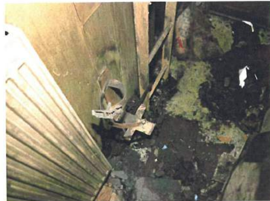
Photograph 29. Fire extinguisher holder at the corridor between the crew cabins.
