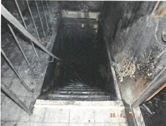
Photograph 8: Stairs leading from the main deck to the crew accommodation
