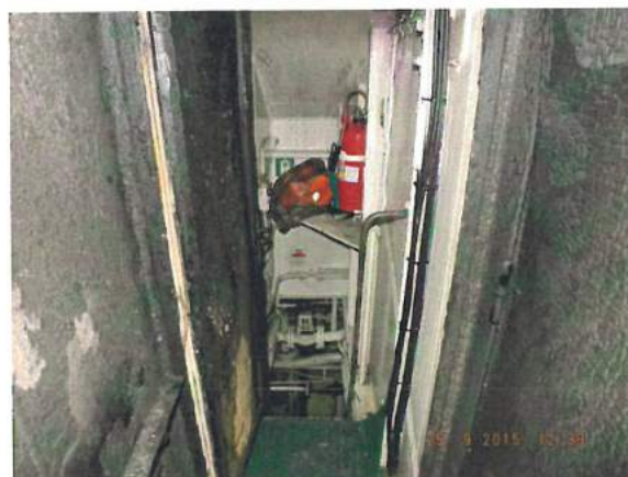
Photograph 27: The entrance to the engine room
