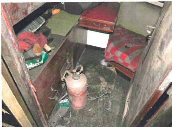
Photograph 28. Fire extinguisher found in the first cabin (from the bow) at the port side.
