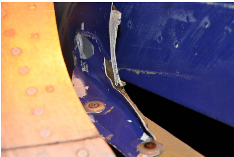
Photo 11: Failed part of fairing still attached to A/C with screws NAS1203-6 and (out of sight) bolt NAS1203-3
