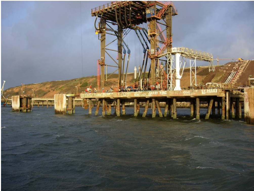
Fig 1. SemLogistics pir nr 2, Milford Haven
