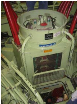
Assembly as original (cover taken off) above pod room deck.
