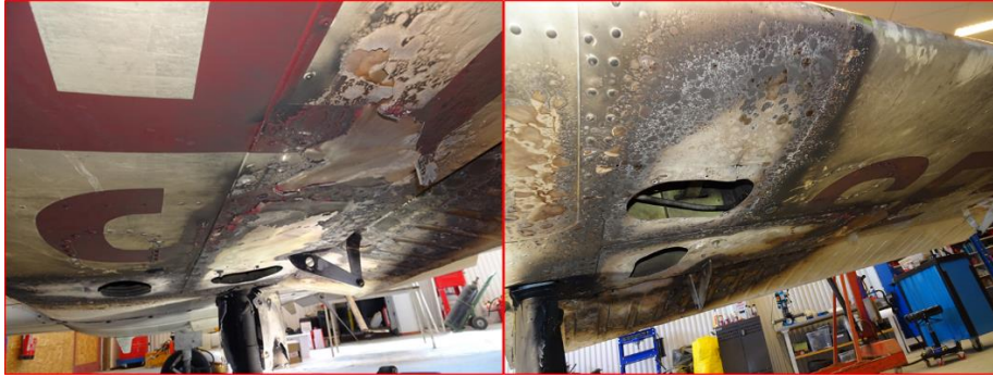
Figure 13. Pictures on the underside of the wing that had been ravaged by fire.
