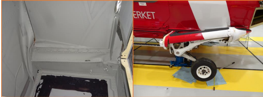
Figure 14. Right image: The damaged main landing gear and surrounding structure. Left image: Structural damage from the inside of the fuel compartment.
