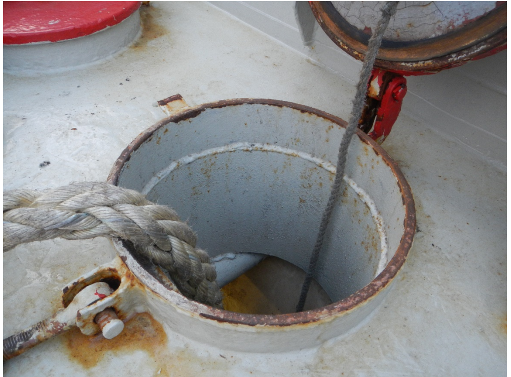
Figure 11. Opening to storage for loose ropes.
