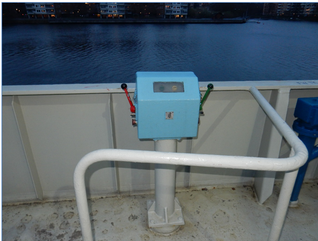
Figure 16. Control box for the mooring winches on the portside bulwark.
