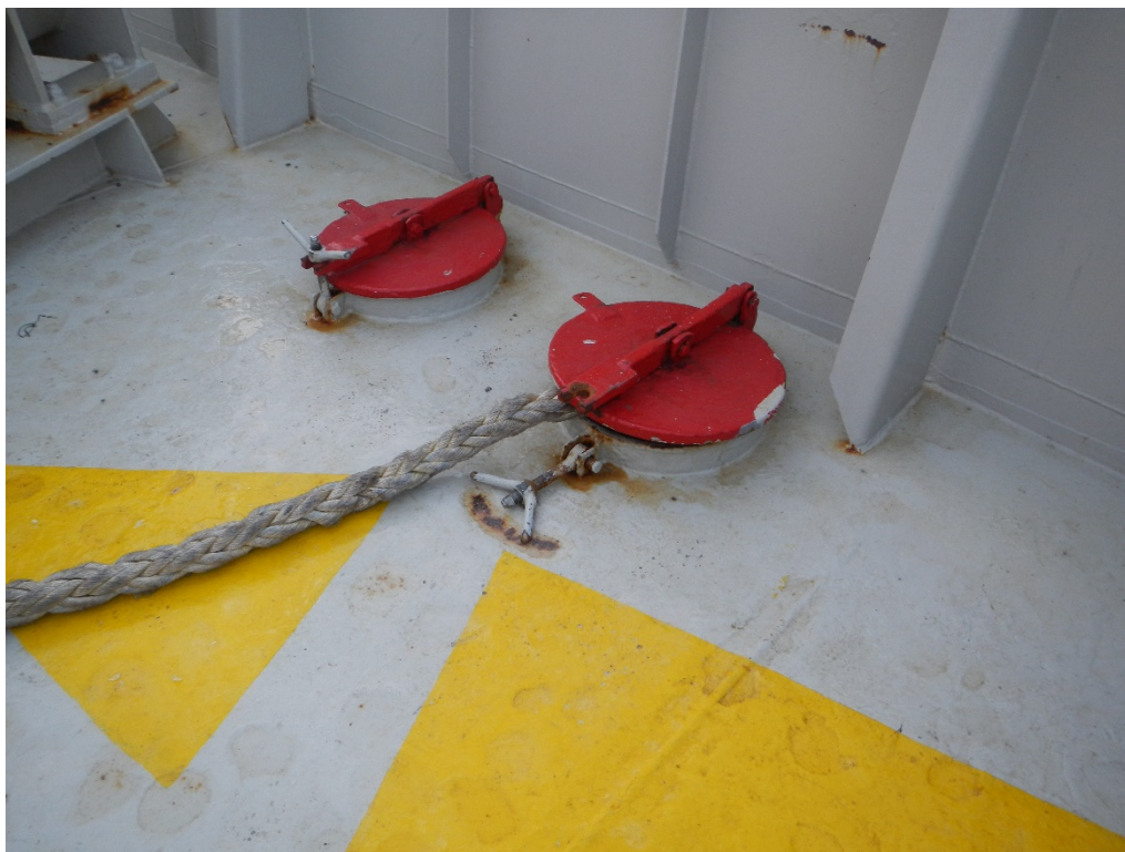
Figure 10. Hatches to storage for loose ropes.
