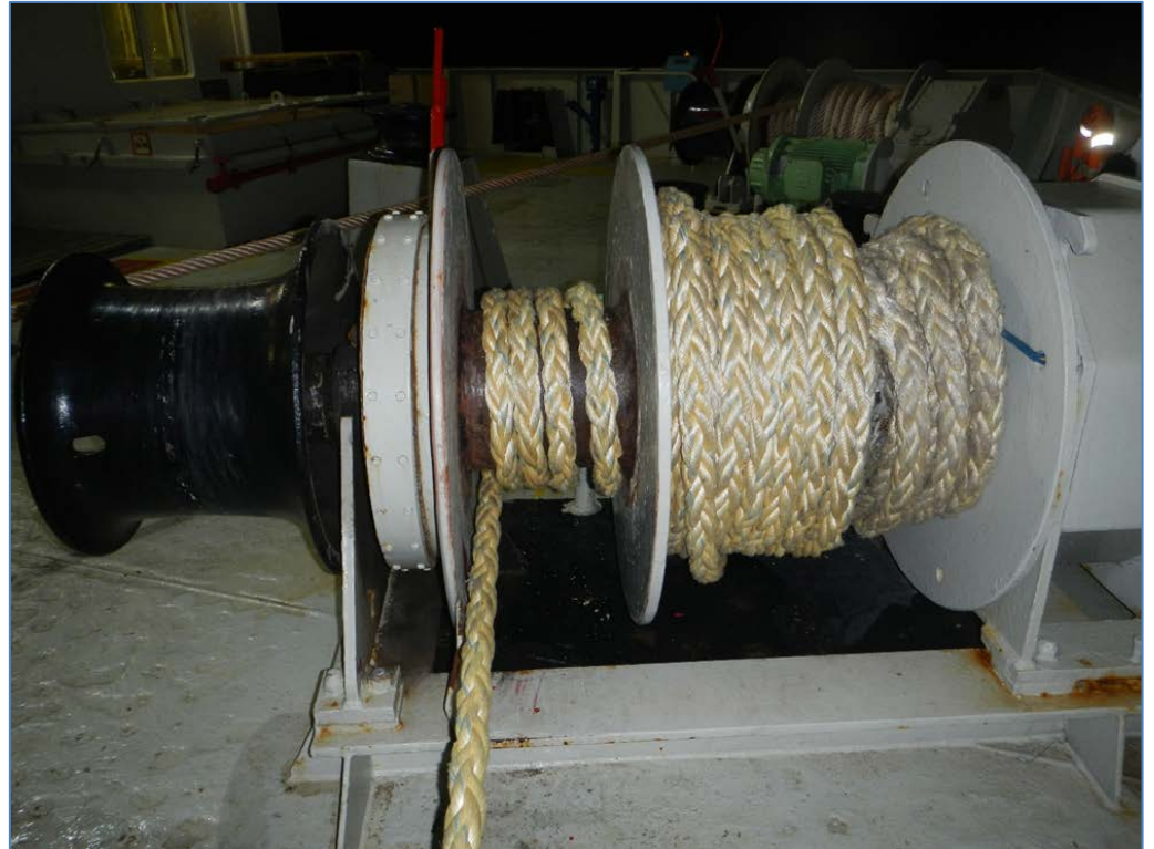
Figure 14. Mooring winch – the regular mooring line running from the loadbearing drum of the winch.
