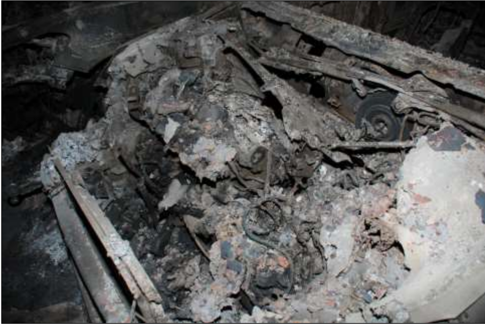
Figure 111: Car 4 B (the car destroyed by the fire most severely and thus the most likely location of the seat of fire)
