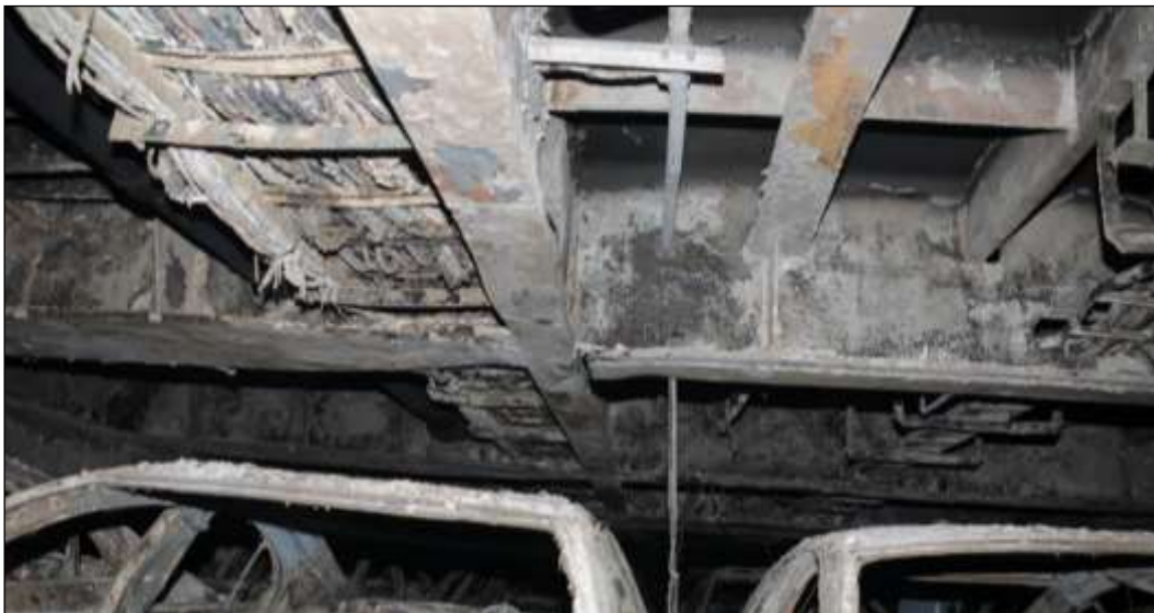
Figure 5: Effect of fire on the cargo hold ceiling and cable routing
