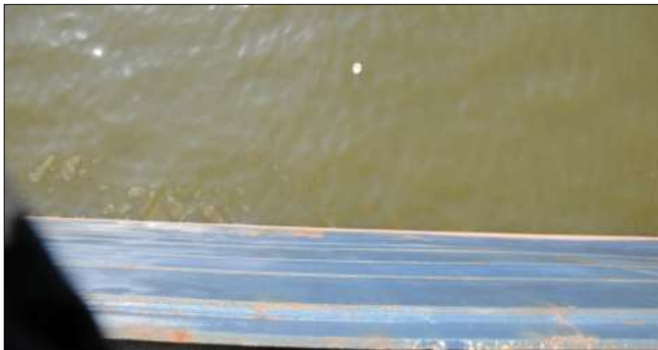
Figure 58: No thermally induced damage to the hull wall in the area of bay 26 (port side)
