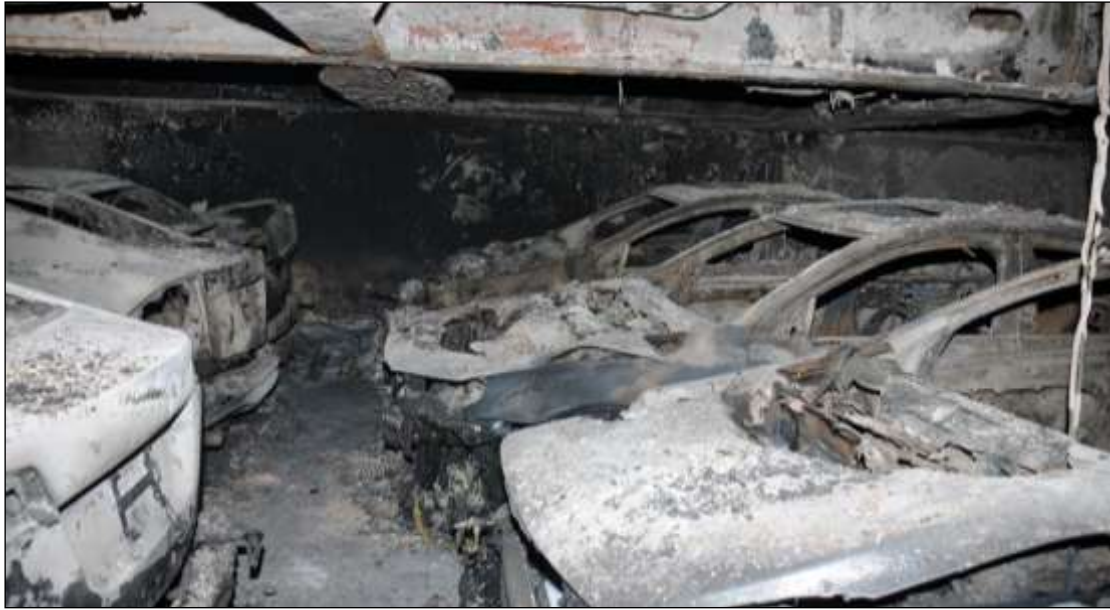
Figure 7: Completely burnt out vehicles on deck 3 B
