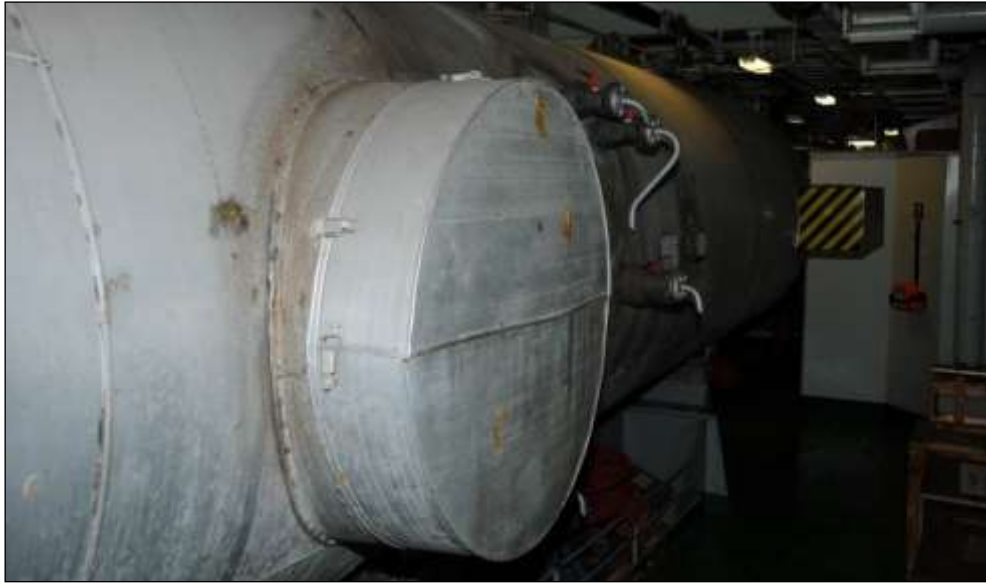
Figure 16: CO 2 low-pressure tank
