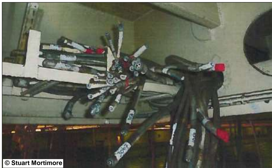
Figure 82: Cable marked for repair purposes 55
