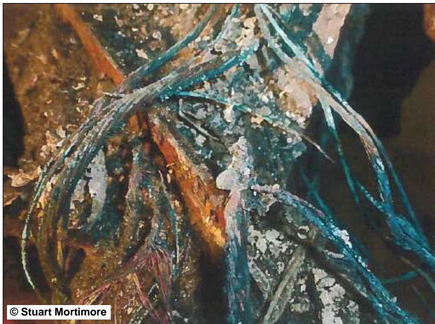
Figure 103: Example of arcing activity caused by electric current (2) 76
