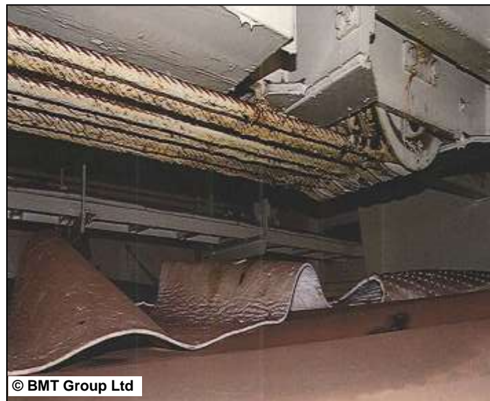
Figure 76: Close-up of a tarpaulin with layer for absorbing fluid
