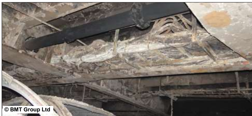
Figure 61: Cable splices on the ceiling of vehicle deck 3 B 34
