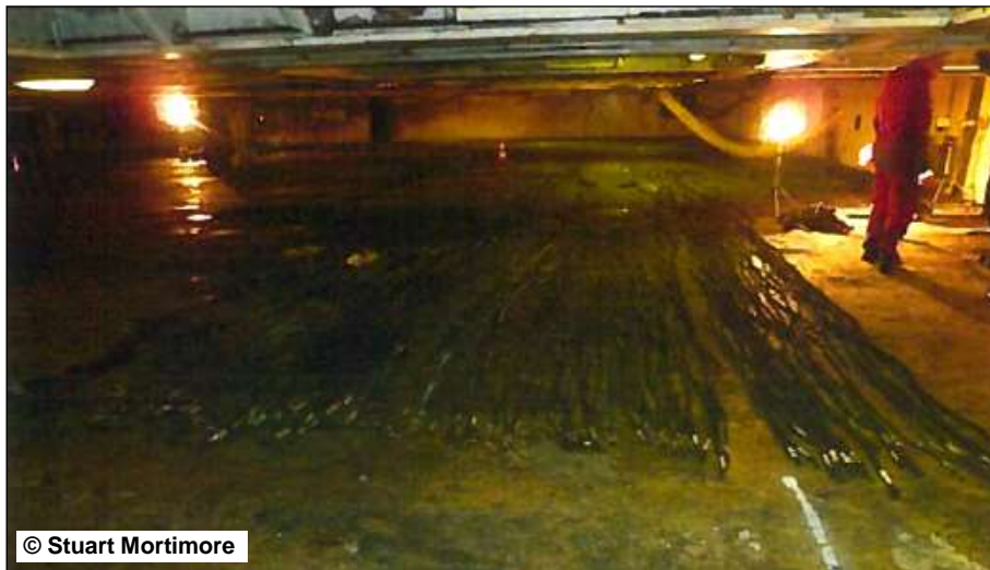
Figure 79: Example of dismantled cable harnesses 52
