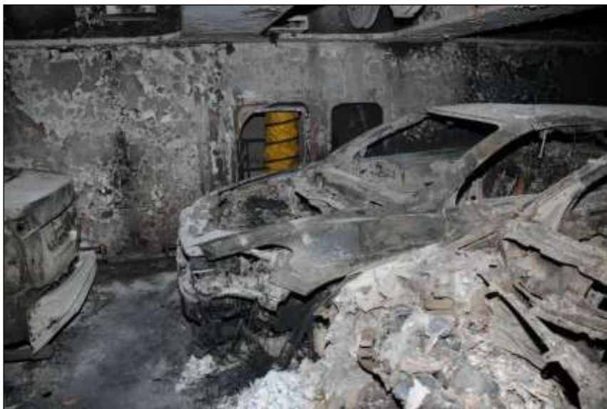
Figure 45: Position of the seat of the fire
