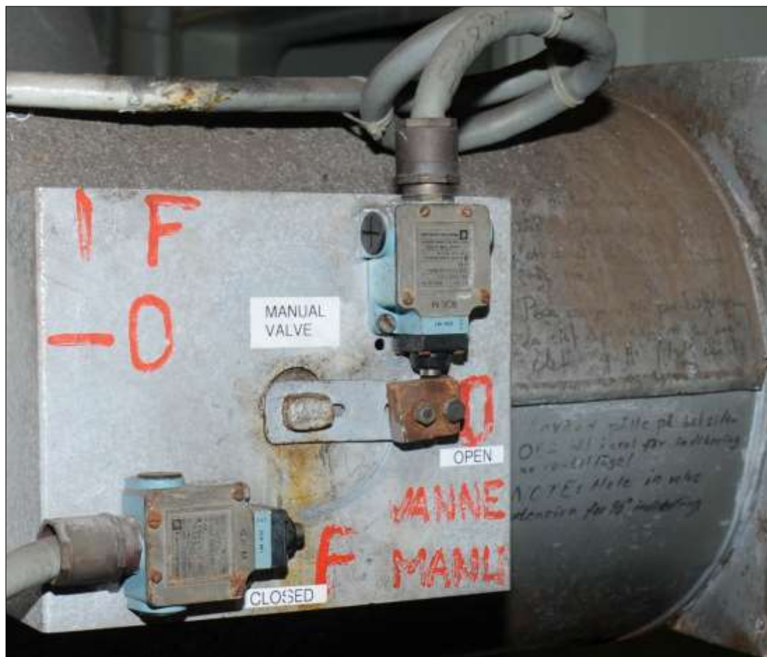
Figure 34: Main tank valve with handwritten operating instructions
