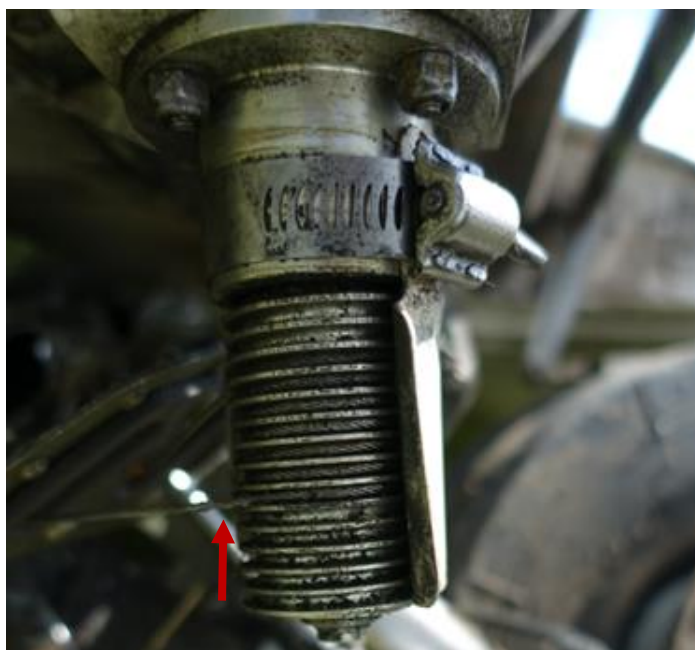
Figure 32. Elevator trim cable position and connection on the cable drum.
