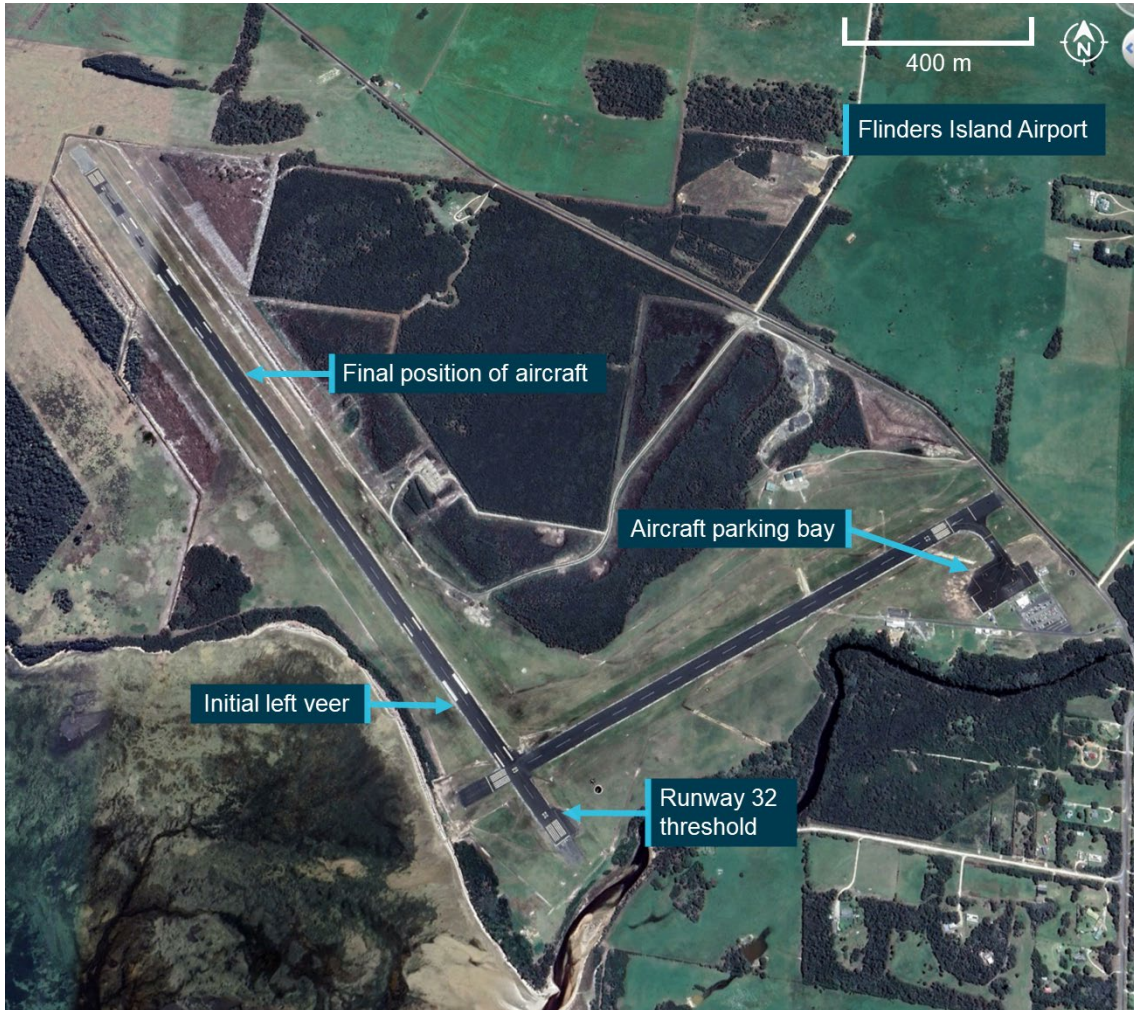
Figure 1: Flinders Island Airport
