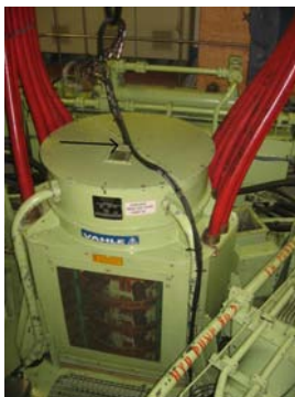
Final assembly. Cables coming through a pipe in center and continuing to the control units.
