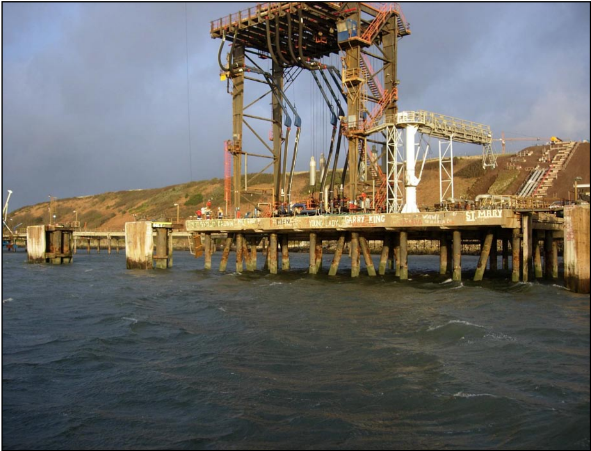
SemLogistics jetty No.2, Milford Haven
