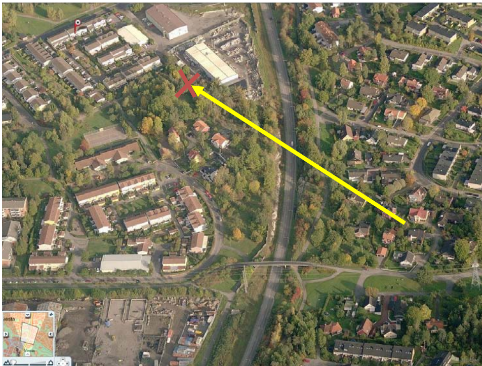
Figure 8. Photograph of the accident site
