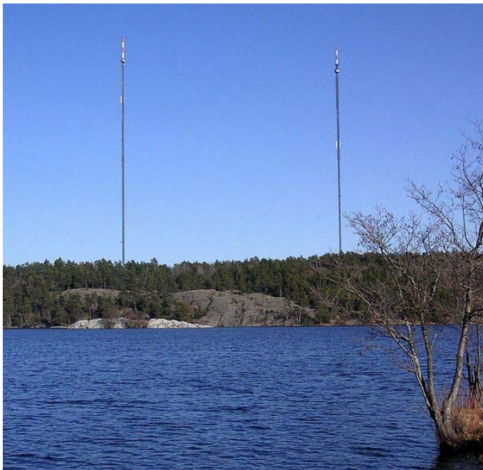
Fig. 1. Radio/TV-broadcasting antennas in Nacka.
