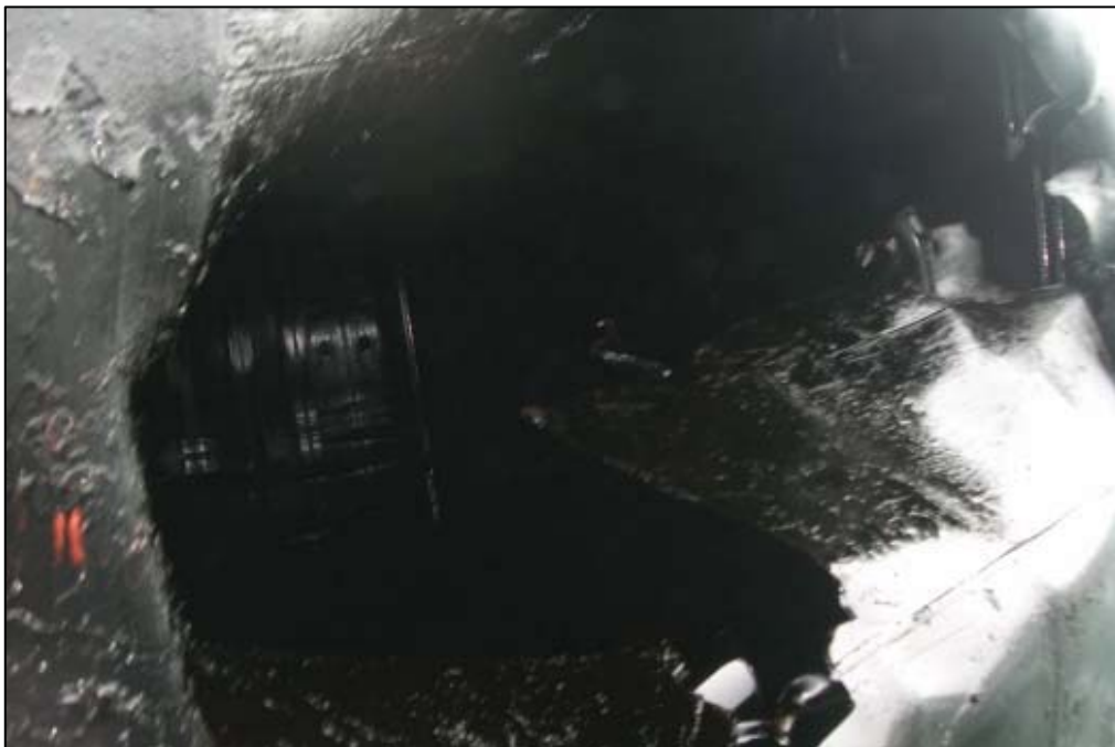
Figure 2: Breached hull i.w.o. no. 1 starboard side heavy fuel storage tank
