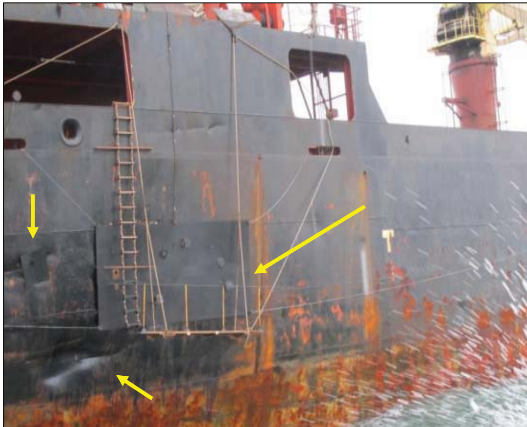
Figure 4: Temporary repairs i.w.o no. 1 starboard heavy fuel oil storage tank
