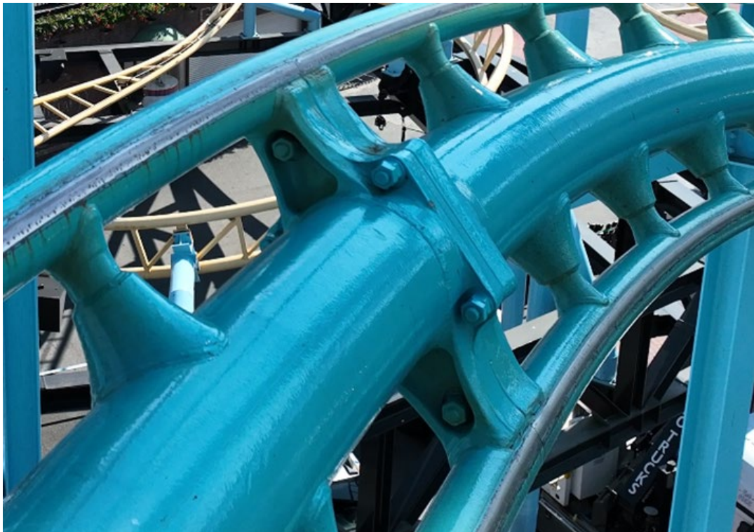
Figure 6. Two track segments and the joint where they are bolted together.
