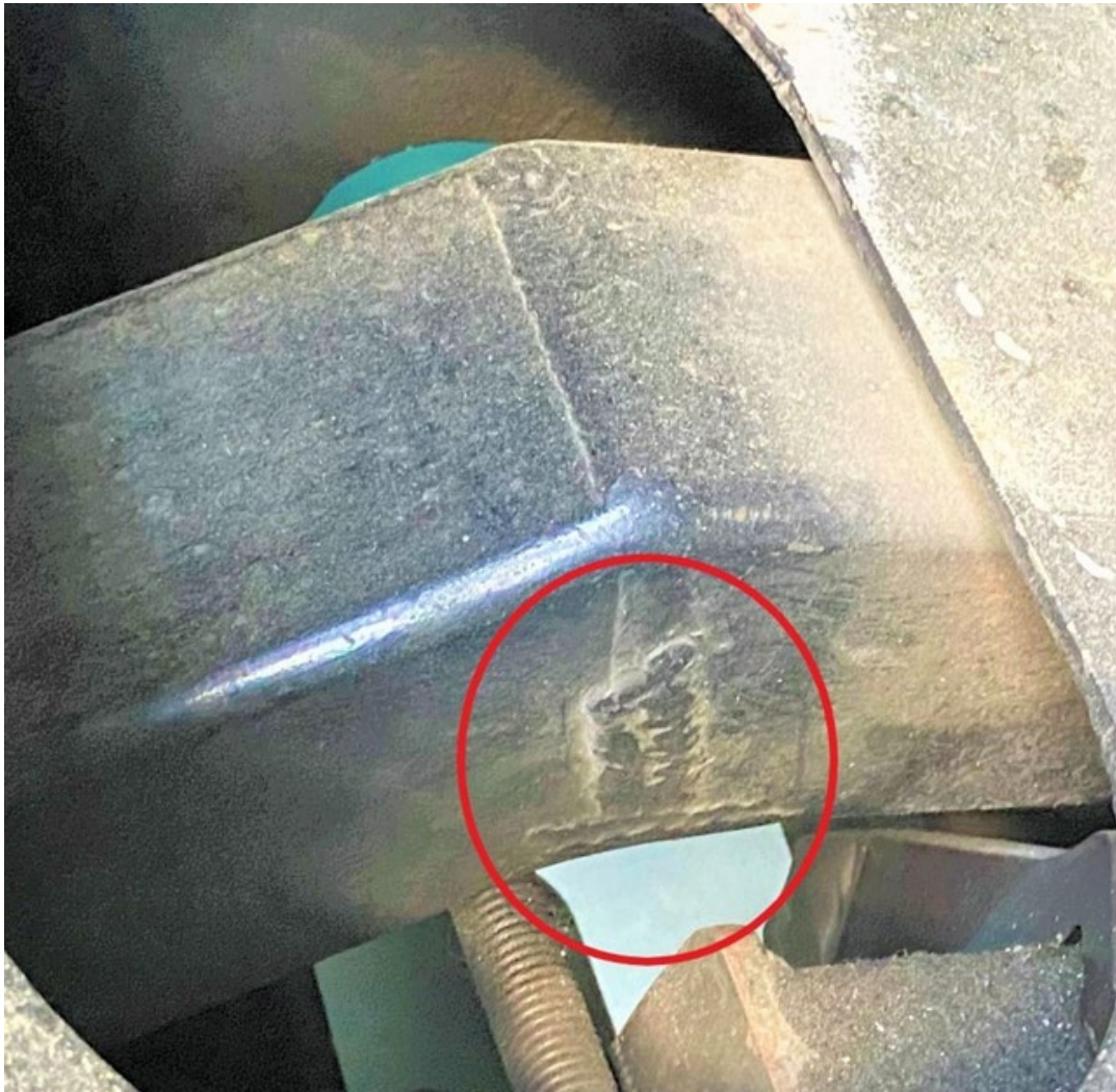
Figure 29. Weld repair on a control arm marked with a red ring. The photo is of a control arm installed on train C. The weld repair is on the weld between the outer and middle parts of the control arm.
