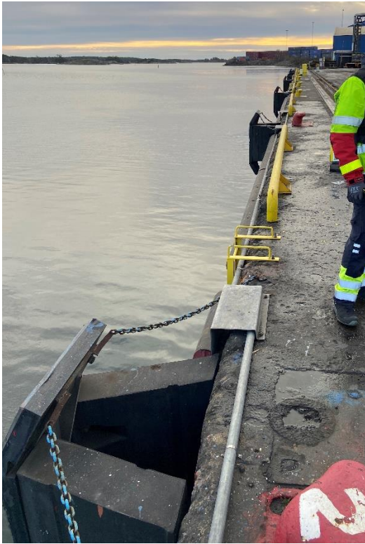
Figure 4. The quay at the steel port in Oxelösund where the accident took place.
