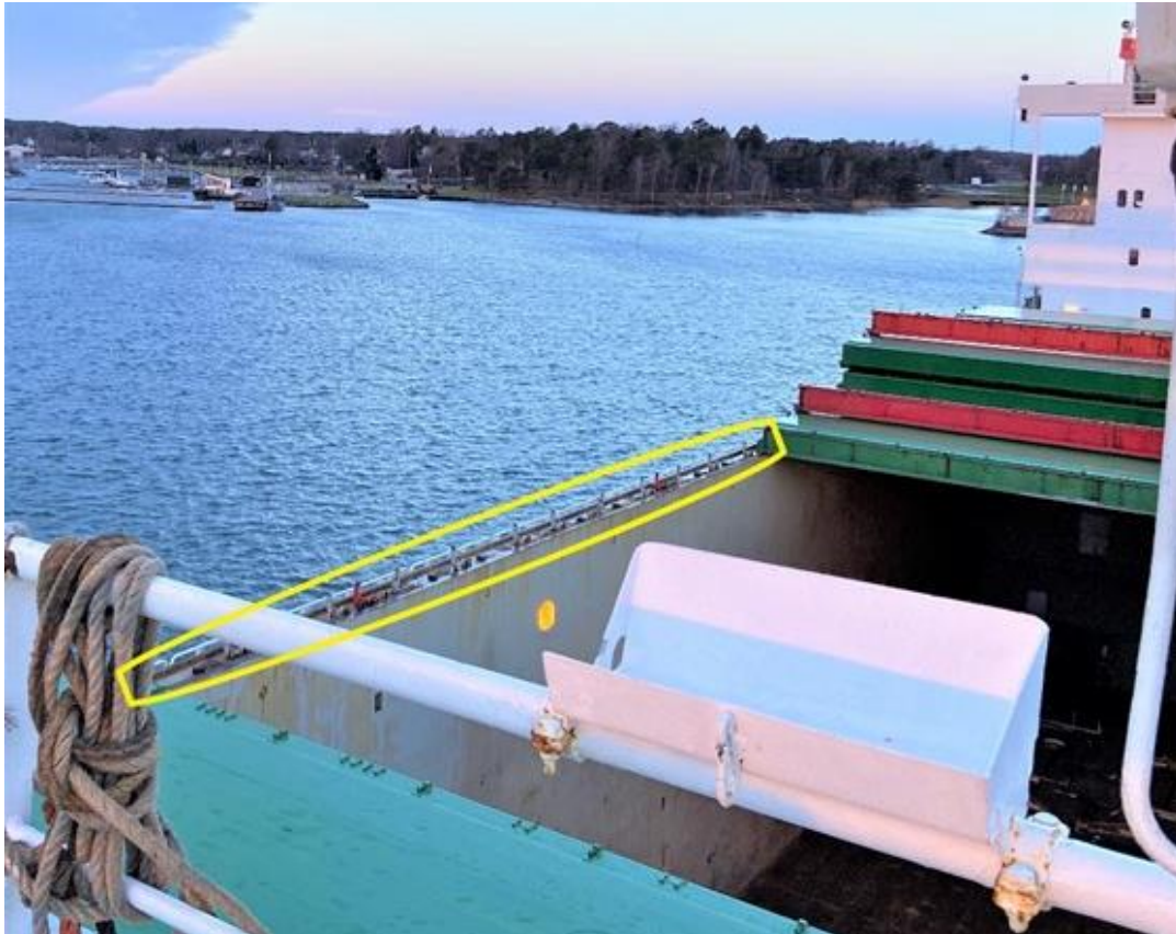
Figure 2. View from the top of the gantry crane. The cargo hold is open and the cargo hold hatches are lying in the background stacked on top of one another. The cargo hold frame is visible within the circled area.
