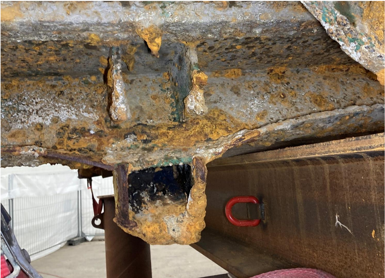
Figure 4. Port side lower ramp side lock box.
