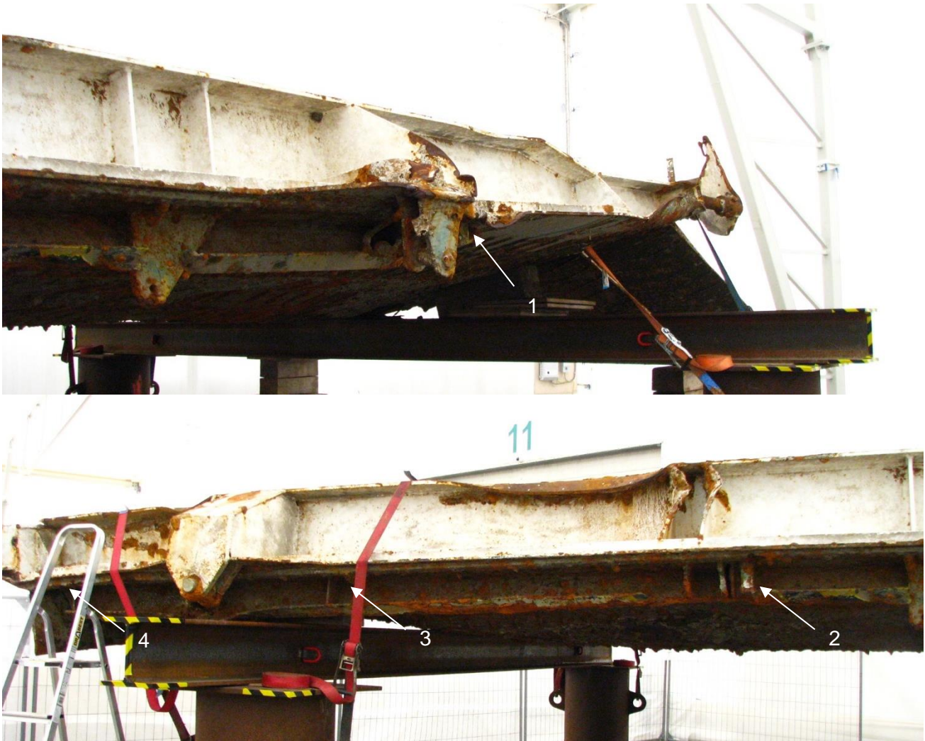
Figure 12. Four attachment positions for railing on the port side.
