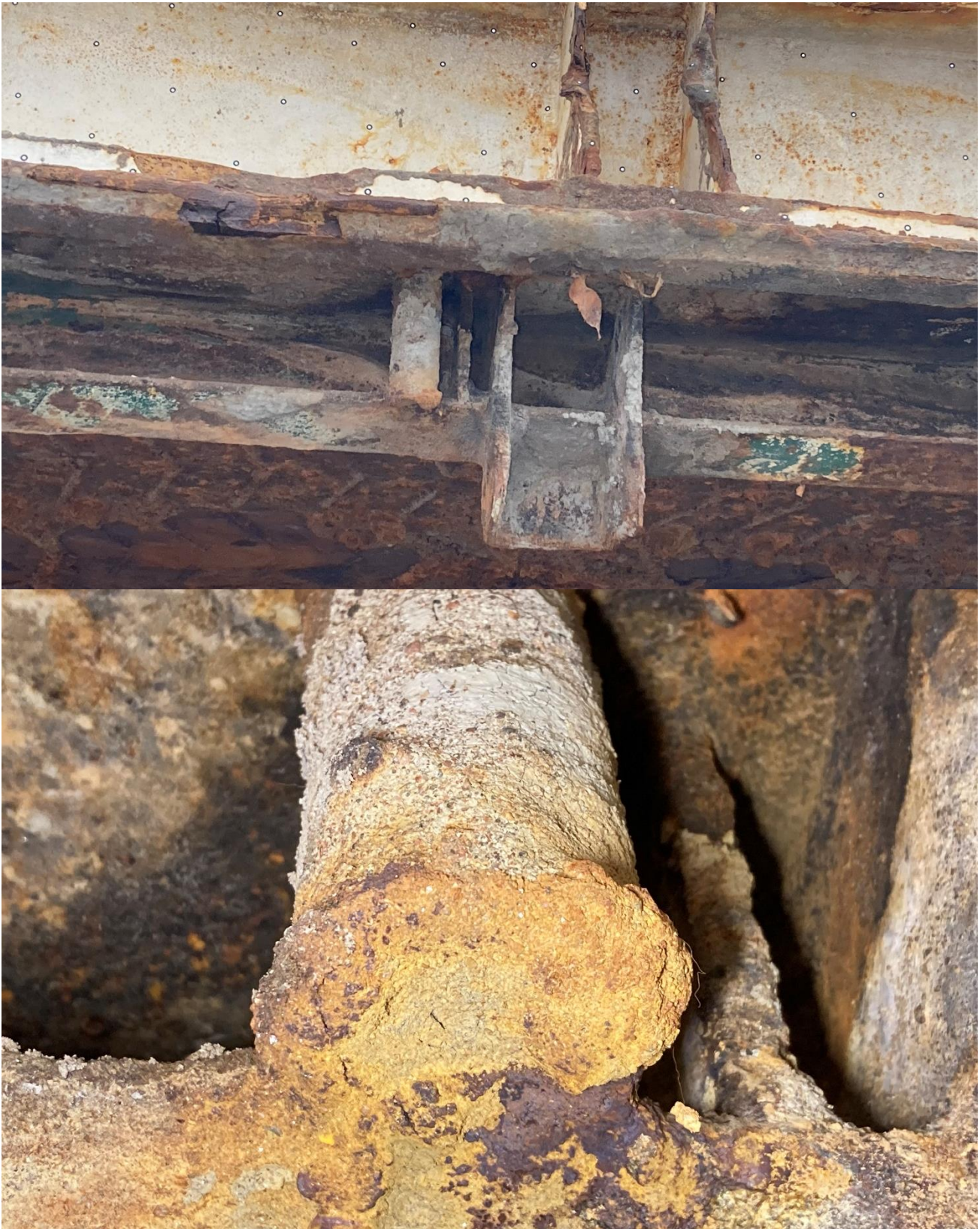
Figure 10. Starboard attaching position for railing (2 in Figure 8).
