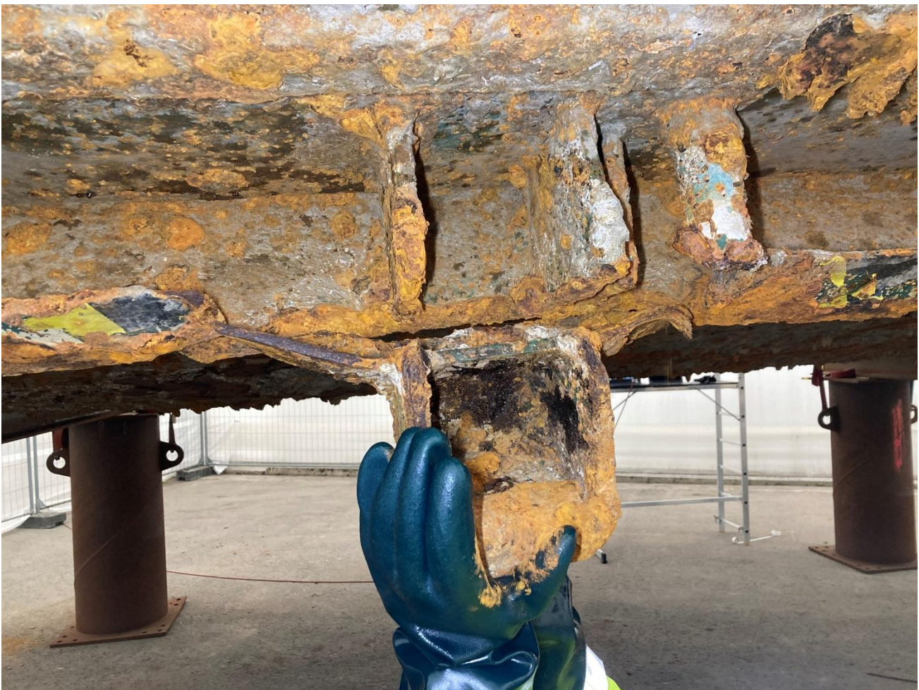
Figure 3. Port side upper ramp side lock box.
