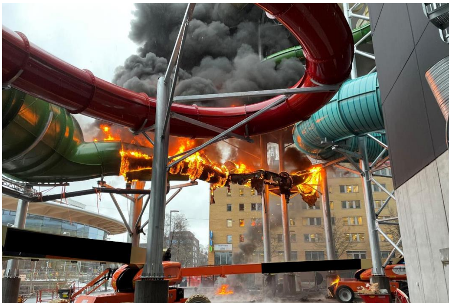
Figure 7. Picture taken at 10:11 hrs, six minutes after the first flames emerged from Rattler. Photo: Sweco AB.
