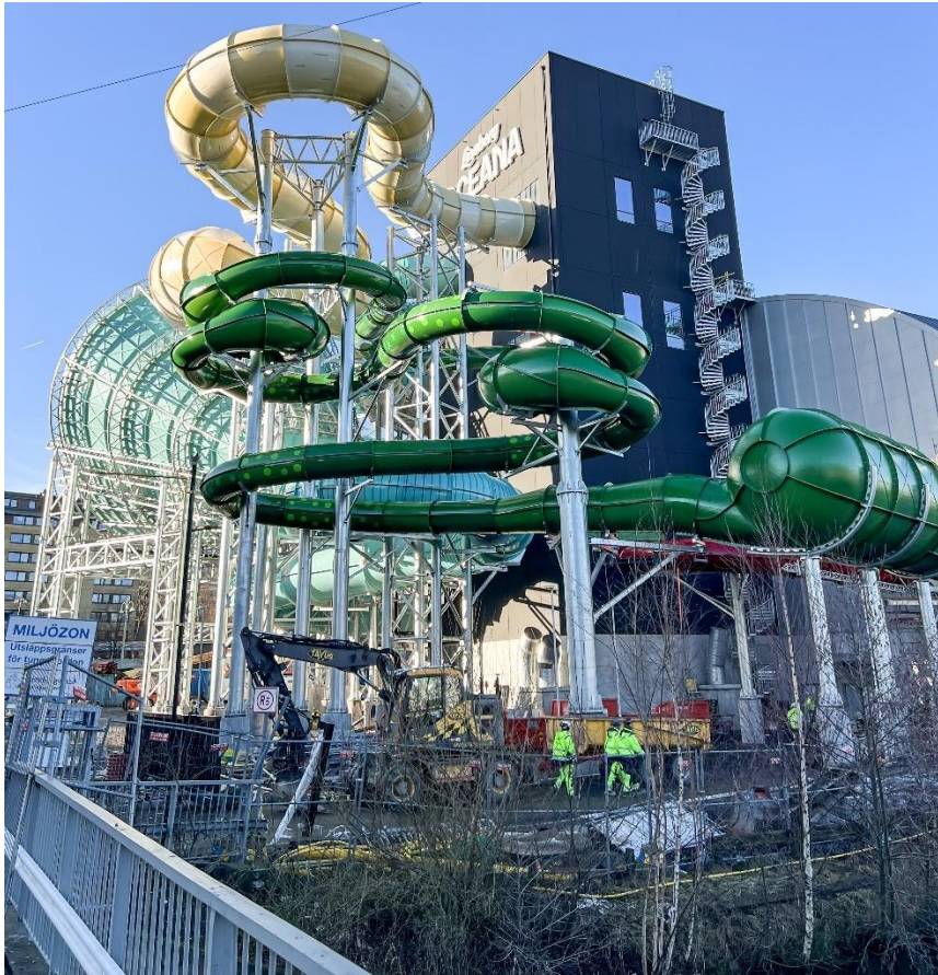
Figure 3. The image shows the waterslides under construction. The four waterslides started in the tower and ended in the pool building. The waterslide Rattler, which is coloured green, is visible in the foreground of the image. The spiral staircase that was the only way to and from the technical space on the top level (level six) is also visible. Photo: Enviro-Process Sweden AB.
