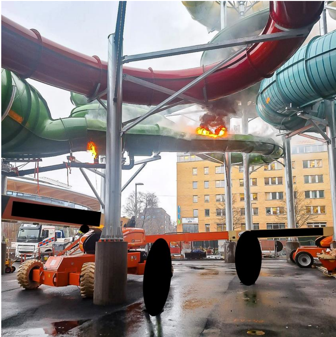
Figure 5. Flames emerged from two places on Rattler at approximately 10:05 hrs. People in the picture have been anonymised by SHK. Photo: Tingstad Måleri AB.
