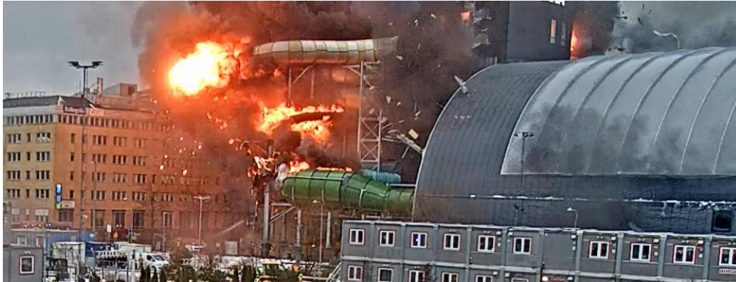
Figure 9. The fire gas explosion at 10:20 hrs. Source: Liseberg.
