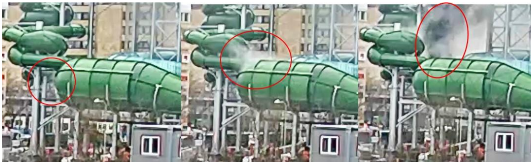
Figure 4. Series of images from a security camera video. Light-coloured smoke can be seen coming from the waterslide Rattler at 10:03 hrs. At 10:04 hrs the intensity of the smoke has increased and at 10:05 hrs it has become darker. Source: Liseberg. The red circles that mark the smoke have been added by SHK.
