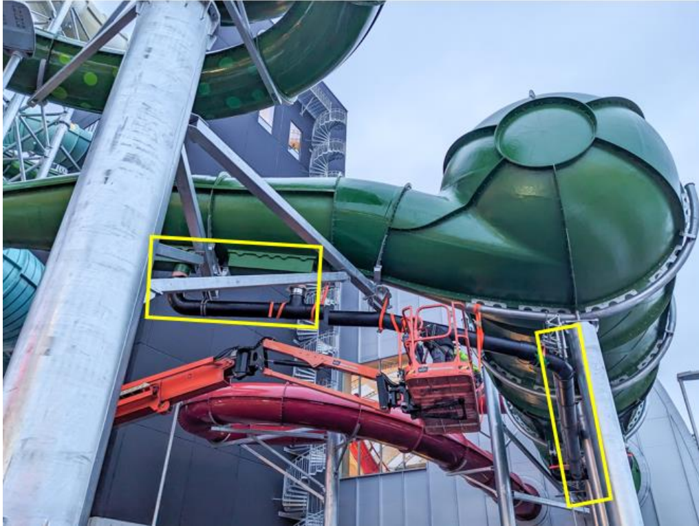
Figure 11. The yellow boxes added by SHK show, on the left, a PE pipe connected to the drainage boxes and, on the right, a PE pipe that connects back to Rattler. A suspended pipe in the strap that has been prepared for being fused together with other pipes is visible between the markings. Photo: NCC.
