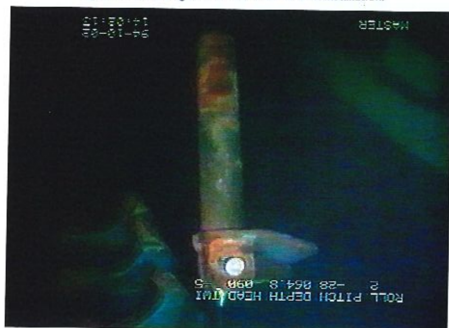
Figure 8.15 Locking bolt for the bottom lock installation.
