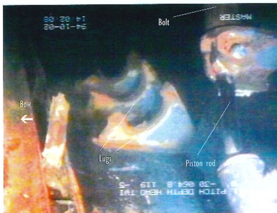
Figure 8.13 Failed bottom lock installation.
