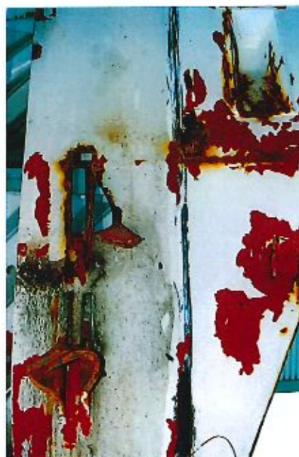
Figure 8.20 Damage on the visor aft bulkhead on the starboard side near the separated side locking lug.
