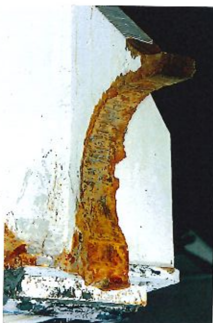
Figure 8.24 Failed starboard lug of visor hinge.
