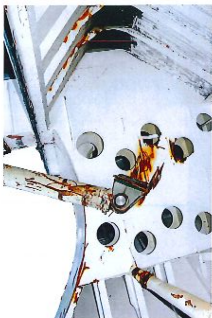
Figure 8.7 Impact marks in the port inner bulkhead, the uppermost cross-bar and the housing on the visor deck.
