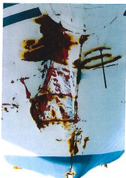
Figure 8.5 Visor damage on the front side.
