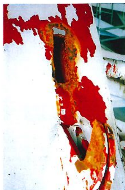
Figure 8.19 Damage due to separation of the port side locking lug, and the lugs of the manual lock.
